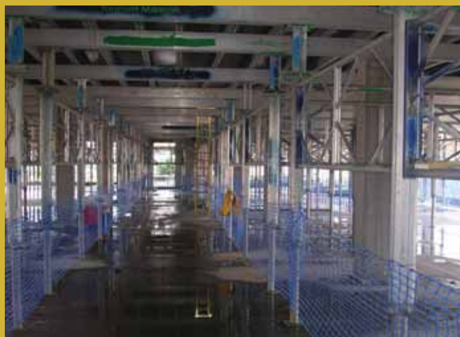
The construction is currently on schedule for the opening in September 2009
